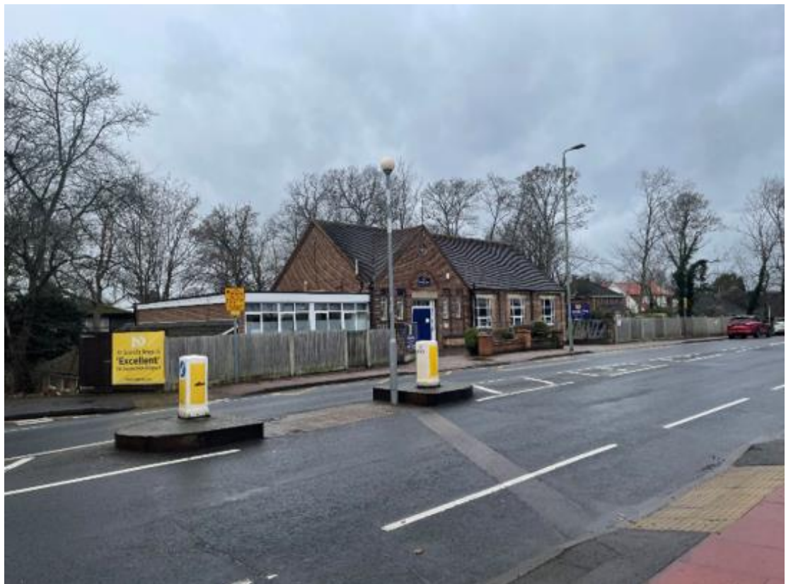
Fig.2 – Site Photo of existing Justin Hall school building
