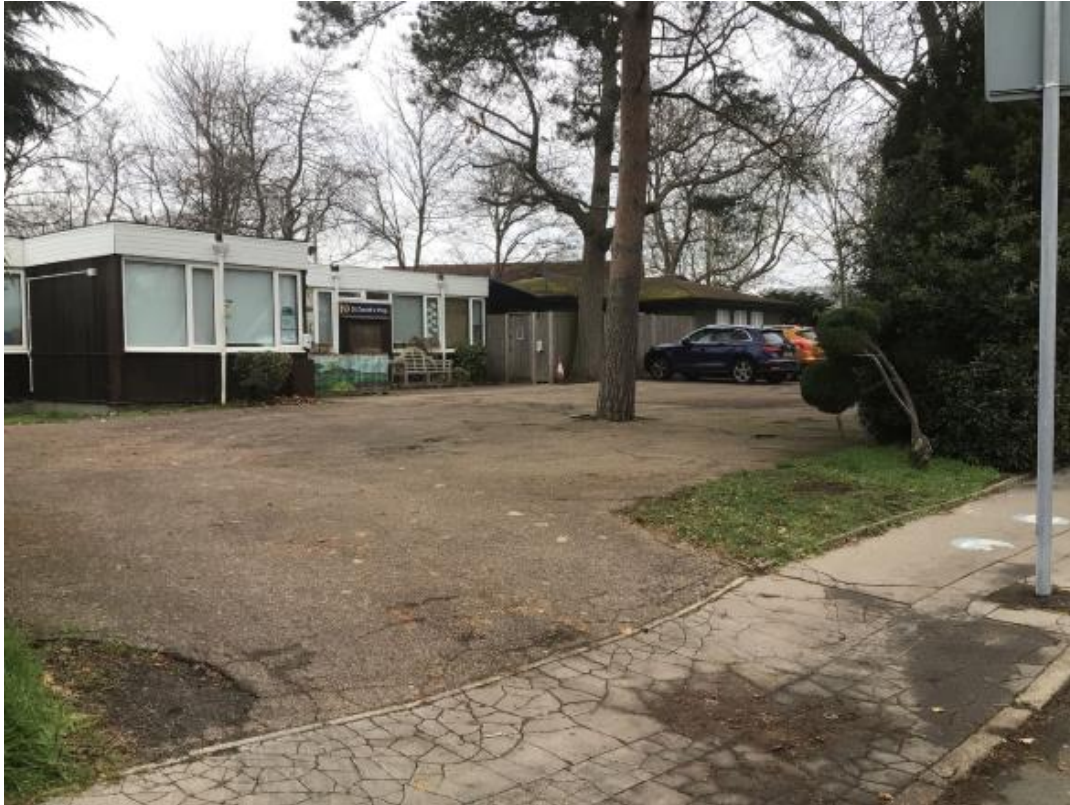
Fig.3 – Site Photo of existing temporary school building on St. Davids Close
